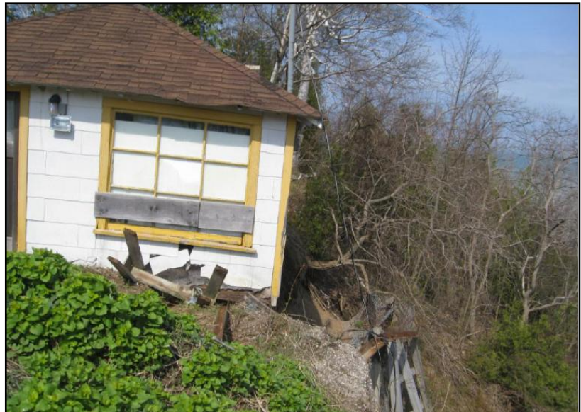
FIGURE 3: GULLY EROSION IN THE MAITLAND WATERSHED (SOURCE: MVCA)
